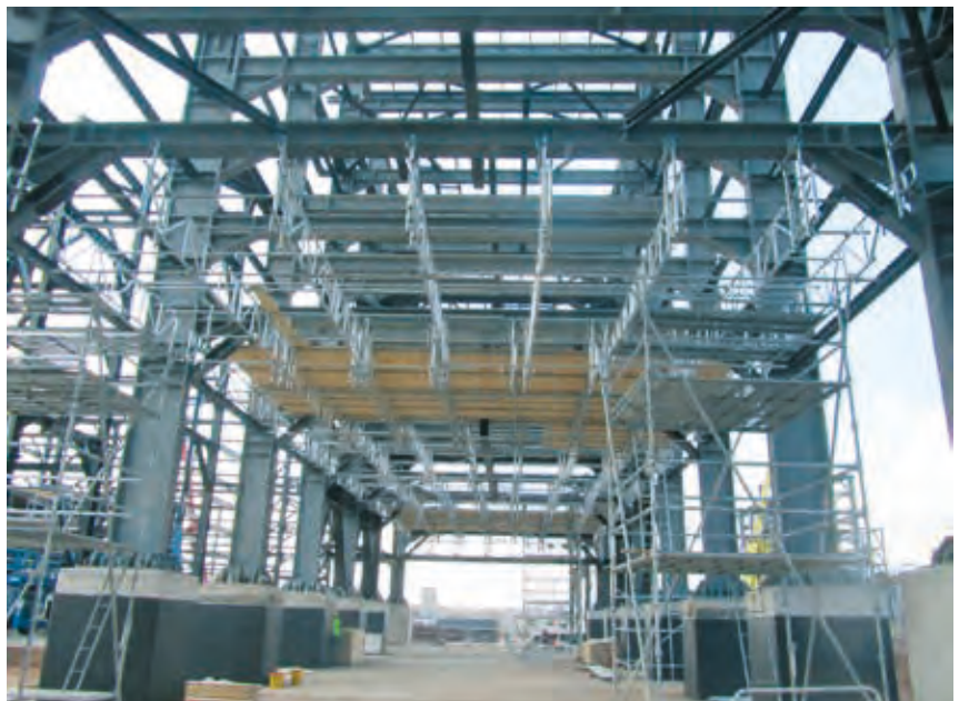
Stair towers provide a safe access with their stable platform and anti-slip stairs.
