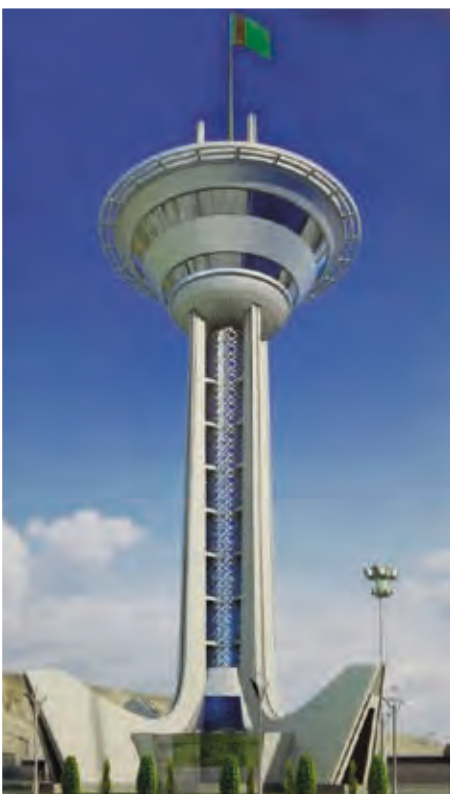
GAP INSAAT, SEAPORT PROJECT / TURKMENISTAN
