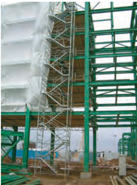
Stair towers provide a safe access with their stable platform and anti-slip stairs.
