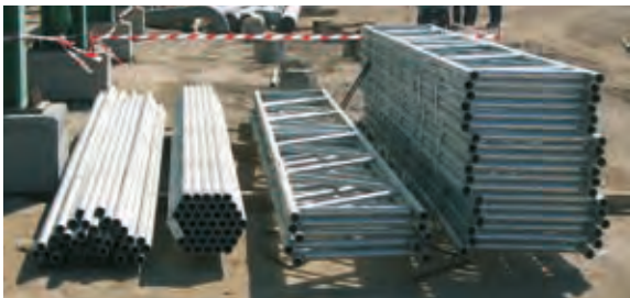
Unit Beams & Scaff Tubes
