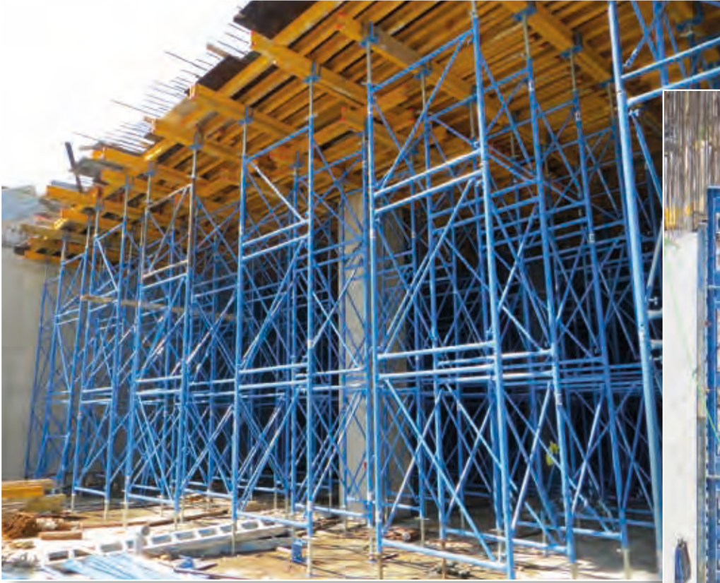
PROMAVI CONSTRUCTION, KARTAL - PENDIK METRO PROJECT/ TURKEY
