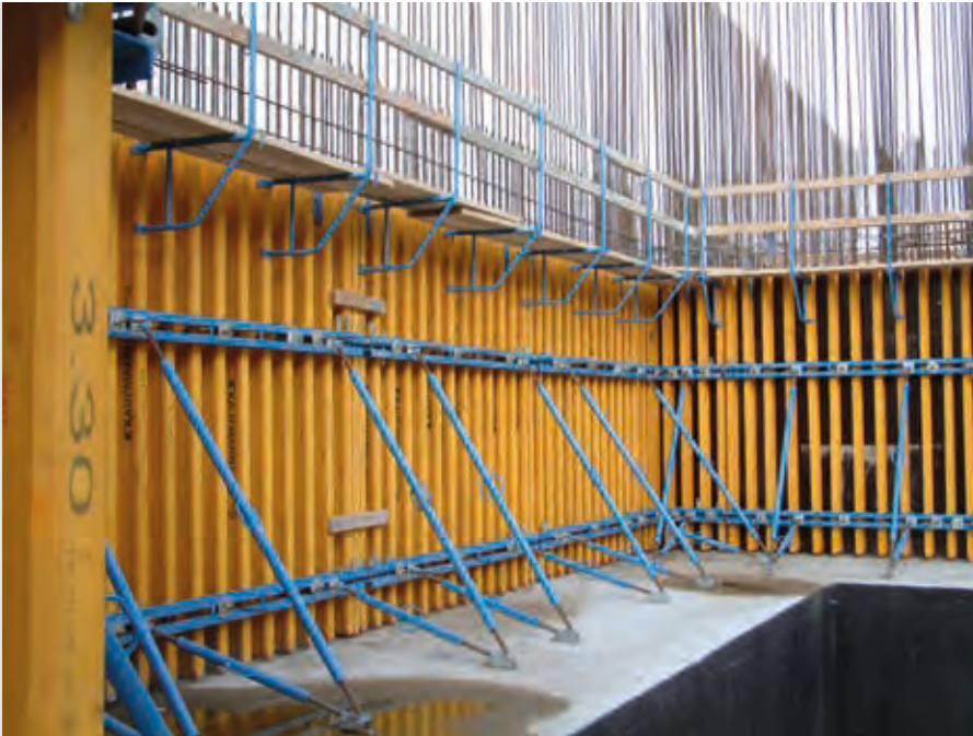
Assembling of the panels in the TMS workshop or even on the job-site.
